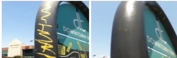
Cleaned graffiti off kiosk at old Chili's
